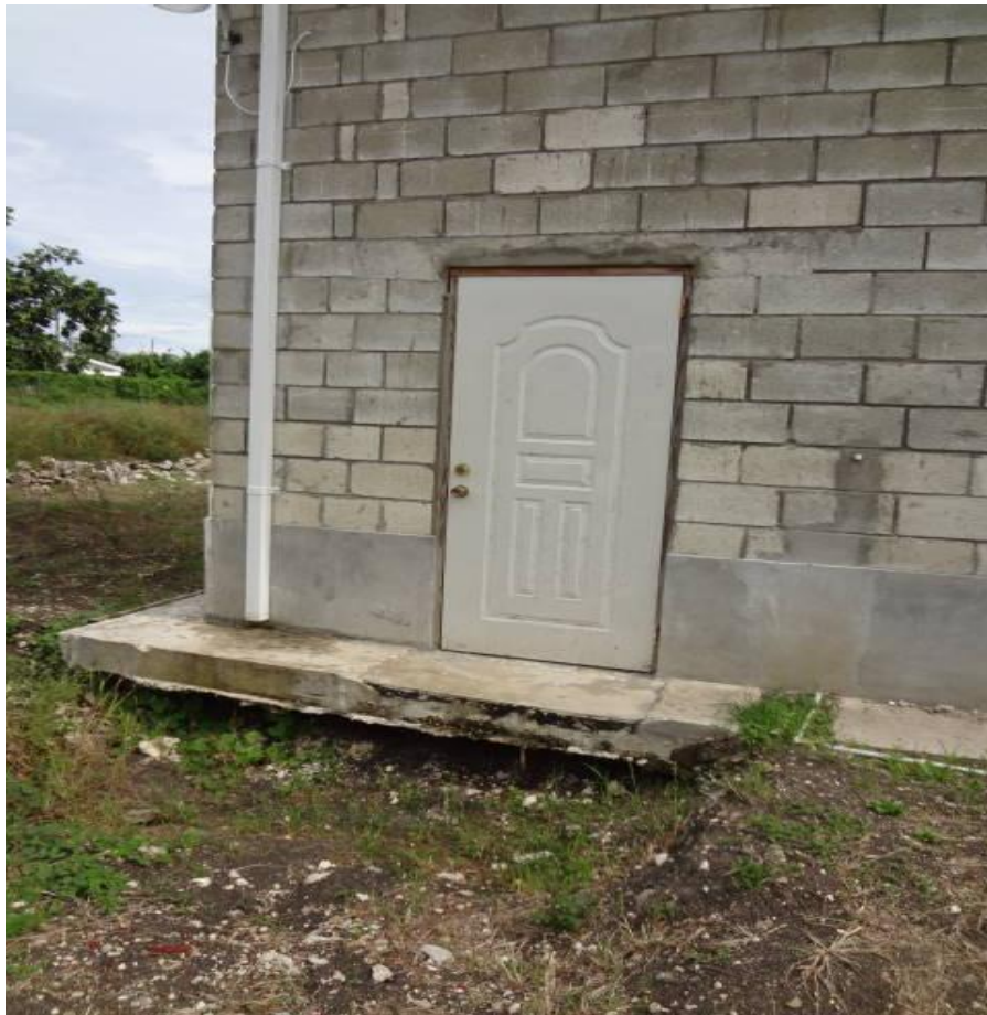
Photo 2: Supporting foundation not buried below the ground surface
