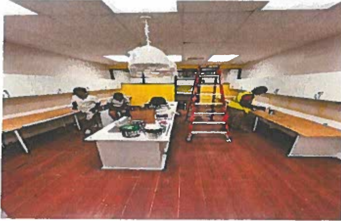
Works in progress
