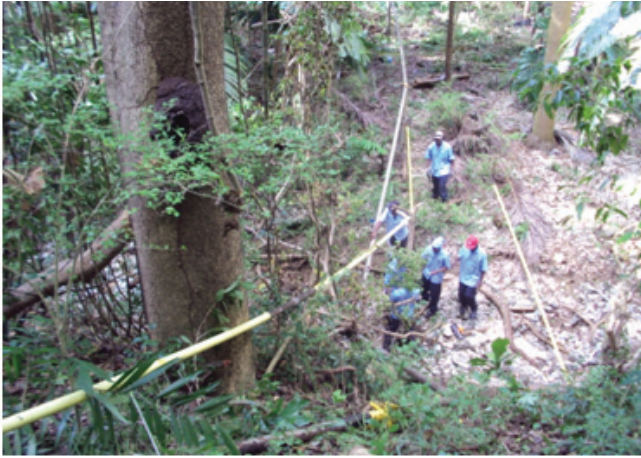
Staff working of Fire Hill Section of Overland Line
