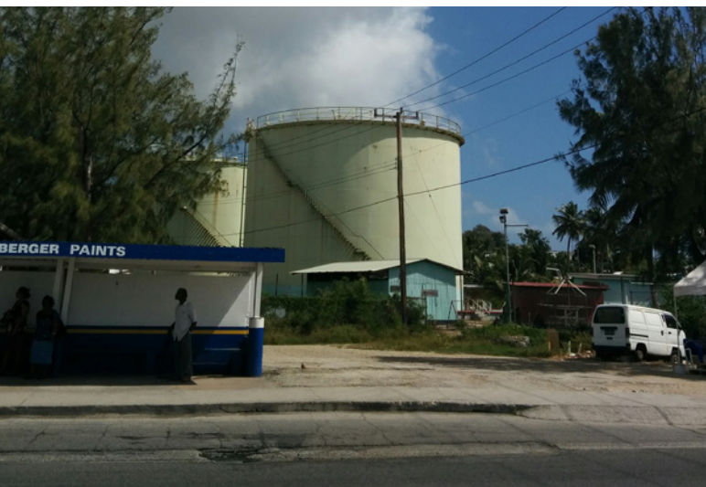
➤ Disused fuel storage tanks, Oistins, Christ Church
