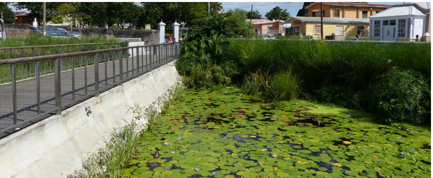
➤ Stormwater Retention Pond, Church Village Green, Bridgetown
