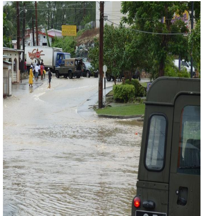
Picture 22: Flooding at Charles Rowe Bridge
