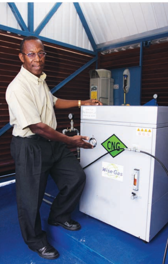
The new Fuelling Station
