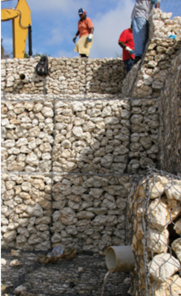
Traditional gabion technology used for road stabilisation programmes in the Scotland District. Photo: Anne Gonzalez
